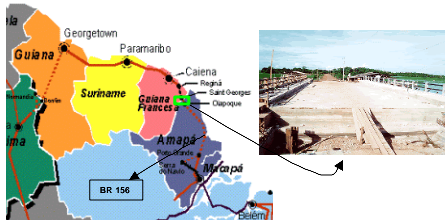
Figure 2.19 Road system connecting Macapá (State of Amapá) to the coastal areas of French Guyana (Caiena), Suriname (Paranaibo) and Cooperativist Republic of Guyana (Georgetown). Picture of Brazil-France international bridge over the Oiapoque River. Source: Rede Brasileira de Centros Internacionais de Negócios ( www.ficr.org.br/cin ) and Government of Amapá.
