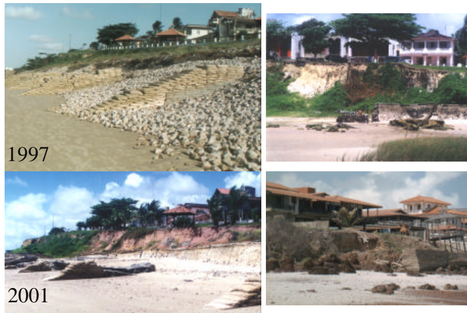
Figure 1.15 Several evidences of coastal erosion on Maçarico and Atalaia beaches (municipality of Salinópolis) affecting high value houses and coastal protection measures.
