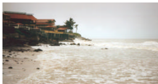
Figure 1.14 The wave power on Atalaia beach (municipality of Salinópolis).
