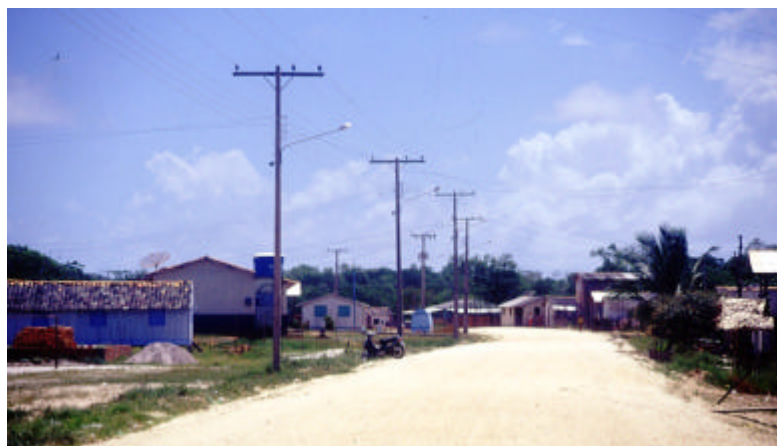
Figure 4.30 View of the main street of Vila Bonifácio, where electric power is supplied to houses, a school and a small hospital.
