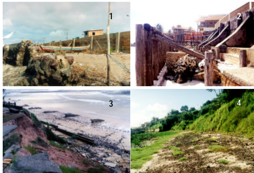
Figure 4.3 Examples show the reduced success of hard structures on the NE coastal area of the State of Pará. (1) Several structures of similar type or little modified in the same area; (2) several structures of different types in the same area; (3) isolated structures, and (4) structures that protect limited areas and increase erosion in adjacent ones.
