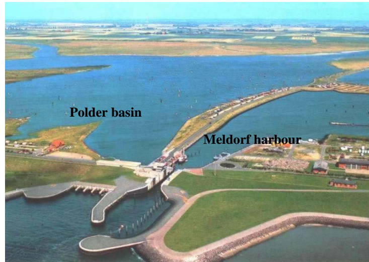
Figure 3.6: Eastern polder basin and the Meldorf Harbour
