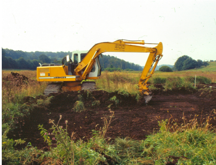
Picture 8. Installation of the three-factorial field experiment in August 2001: top soil removal.
