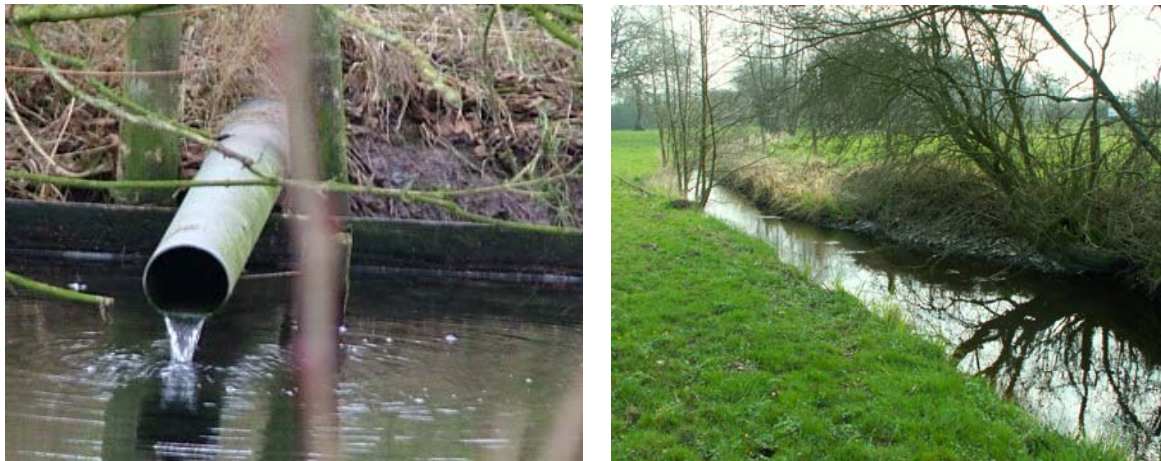
Figure 1.1: Tile drainage and open ditch in the Kielstau catchment (Photo by Bieger, 2007)
