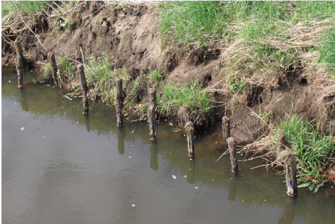
Fig. 5.21 Riverbank erosion in the River Stör at the gauge station Willenscharen (April 2011).
