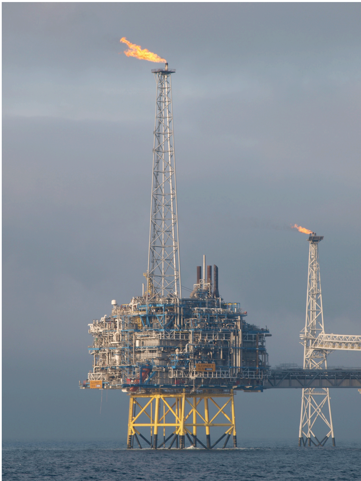
Sleipner CO 2 treatment and injection platform, Norwegian North Sea
