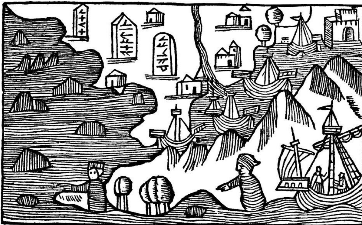
Fig. 4-24. The stone door – porta lapidum – named Hariestic in the Valdemarian Itinerary (near Baggenstället) viewed from the north. Stockholm is depicted on the right side. Not necessarily owed to perspective, smaller vessels are shown entering the southern passage (here: above) and larger take the passage north (here: below) of Wärdö (from Olaus Magnus Historia - 1555, book II, ch. 28).
