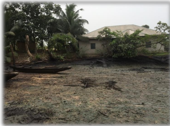
Figure 17: Building of a domestic bourgeoisie @ the background in Ogoni-land, 22.01.2016 (Photo taken by the researcher)
