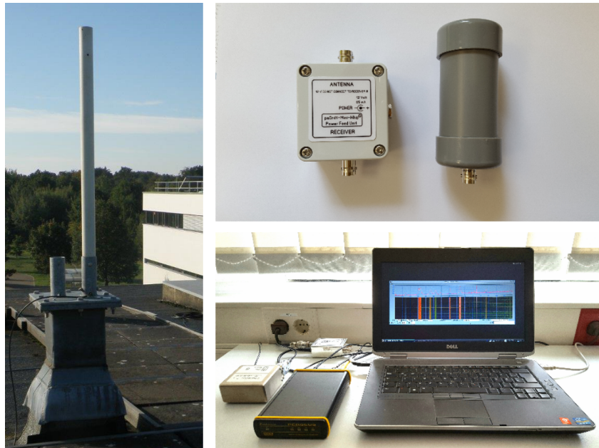
Figure 22: The GIFDS station at DLR Neustrelitz: The left panel shows the set-up of the antenna on the roof. It contains a MiniWhip antenna (detailed view including the remote power supply on the top right). The bottom right picture shows the Perseus SDR receiver. [adapted from Wenzel et al. (2016) ]
