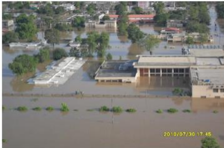
Figure 43: Flood Water in District Nowshera (source: NDMA 2016)
