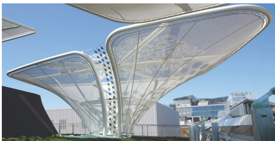
Figure I.6. Solar trees constructed with OPV modules at the Expo 2015, Milan. Adapted from reference. [55] © 2015 S. Berny et al., licensed under Creative Commons CC BY 4.0.
