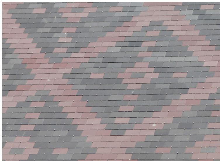
Figure 6. The imported slates (China and Canada) on the Saint Nicolai Church in Plön, arranged in “English” rectangle roofing with hooks (15 years old).
