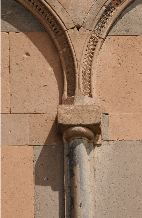
Fig. 13: Ani Cathedral. Fragment of the blind arcade of the southern façade. Photo by A. Kazaryan (2017). All rights reserved.
